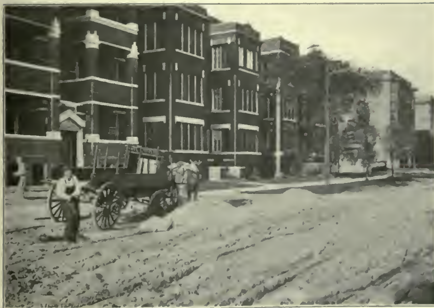
FIG. 36. UNIMPROVED STREET. Photograph taken August 21, 1914. Many of Chicago's streets are unimproved. Constant travel upon them keeps the surface pulverized, and dust from them is easily blown about by the wind.
